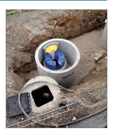
The Hydro Biofilter™ is a biofiltration device that looks like a normal tree or shrub planted through a grate. Underneath, a precast concrete chamber contains a layer of enhanced mulch and a soil filter medium to deliver high levels of surface water treatment before the water is discharged into the drainage system.
