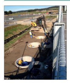
The Hydro Up-Flo™ Filter units will remove fine sediments, hydrocarbons and other pollutants from the car park runoff. They provide a high-performance multi-stage treatment train in a single device by combining sedimentation and screening with fluidised-bed filtration technology.
