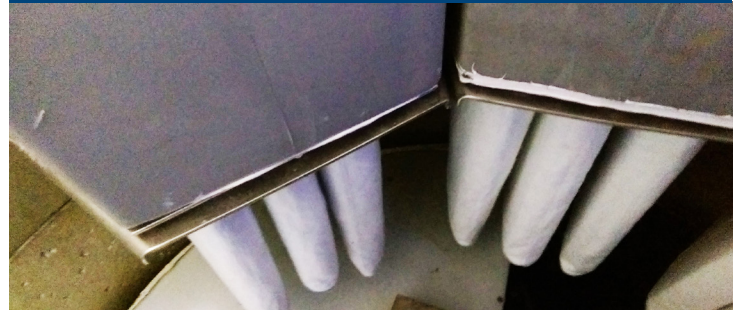
EXTERNAL VIEW OF MEDIA RIBBONS WITHIN A FILTER MODULE
