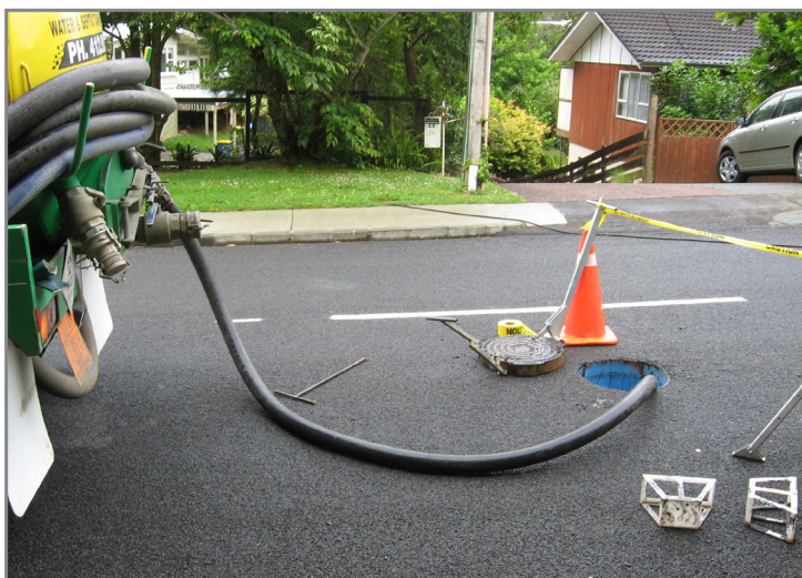
Fig.7 Sediment is removed from the sump with a vector hose. Man entry is not required for this step.
