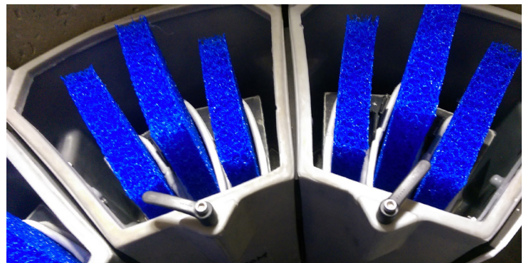
TOP-DOWN VIEW OF MEDIA RIBBONS WITHIN A FILTER MODULE
