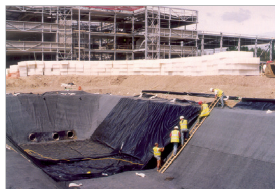
Liner preparation prior to installing Stormcell® blocks
