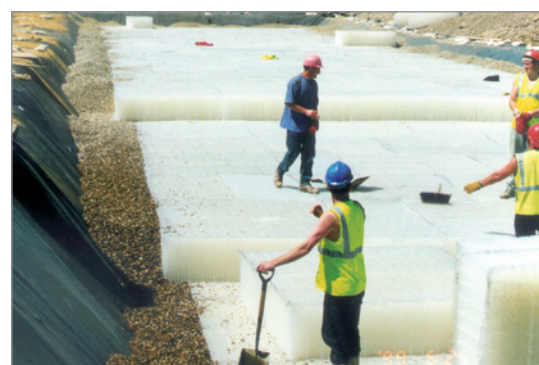
During installation of Stormcell® system
