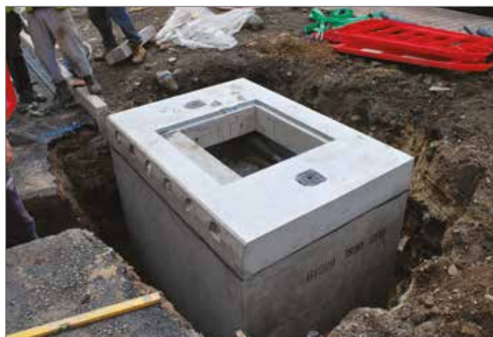
Bungs sealing the kerb inlet slots.
