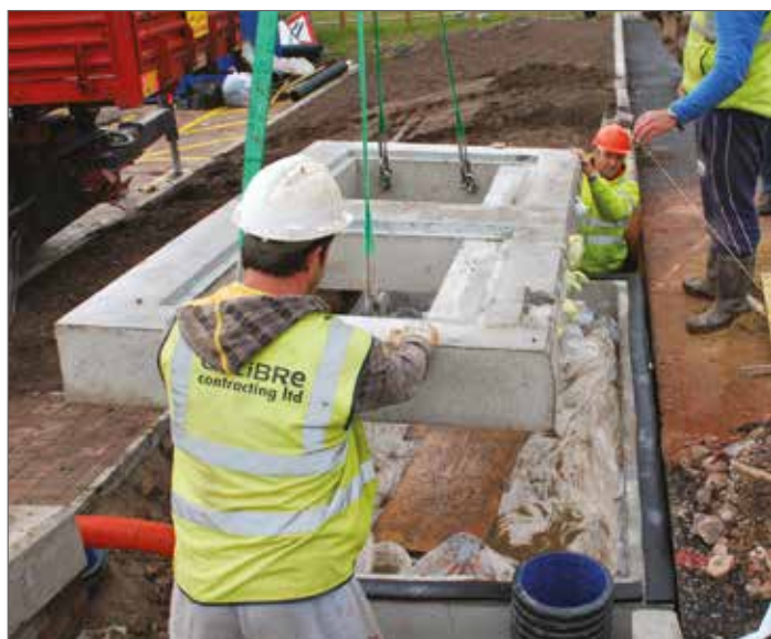
Chamber with Butyl sealant.
