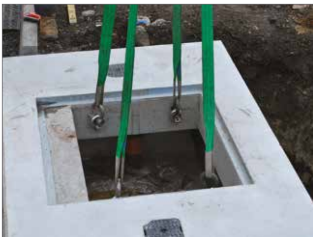
Cover lift and correct lifting points.
