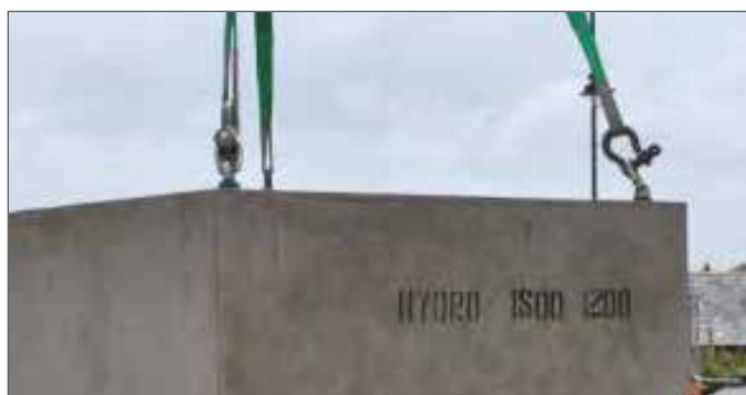
Example of lift and correct lifting points.
