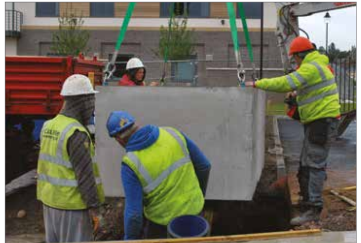
Chamber being lowered into position.
