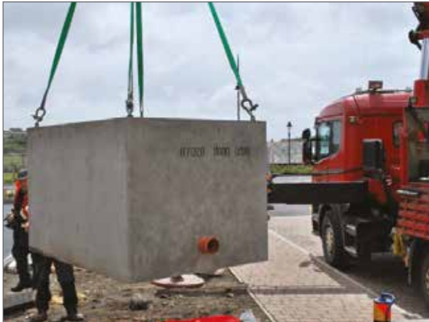
Chamber lift and correct lifting points.
