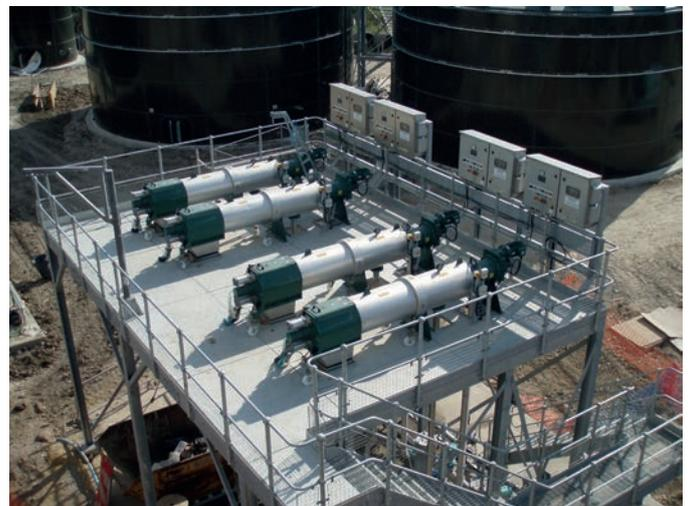
**"The screens operate with three screening and one on standby to minimise any downtime. They are installed on a single concrete plinth, over skips which collect the rag for disposal; their small footprint is ideal for a modern treatment works."**
