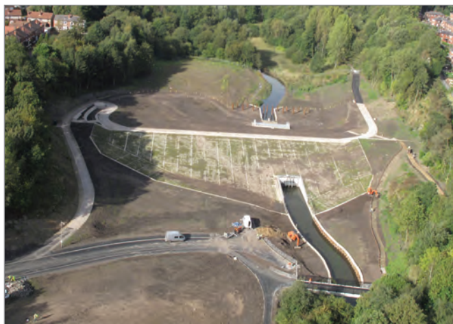
Aerial view during construction.
