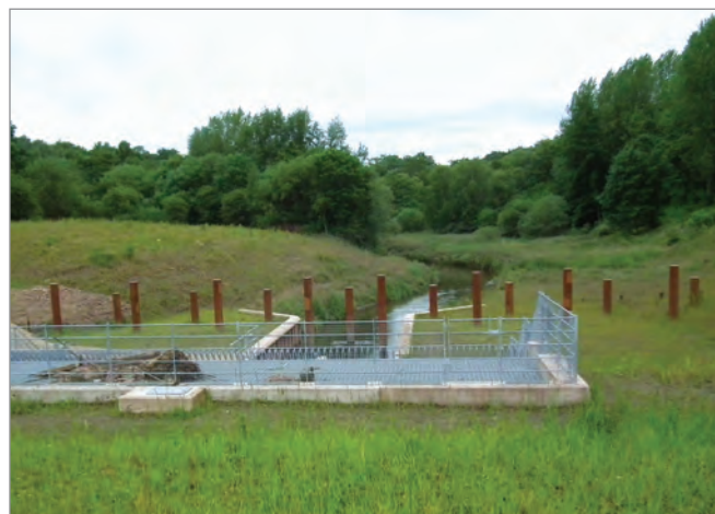
Landscaped area after installation.
