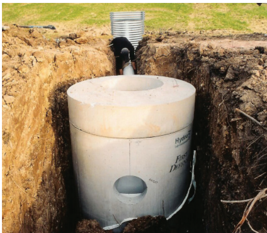
Fig. 1 The First Defense® is delivered to site pre-assembled, facilitating quick and easy installation.
