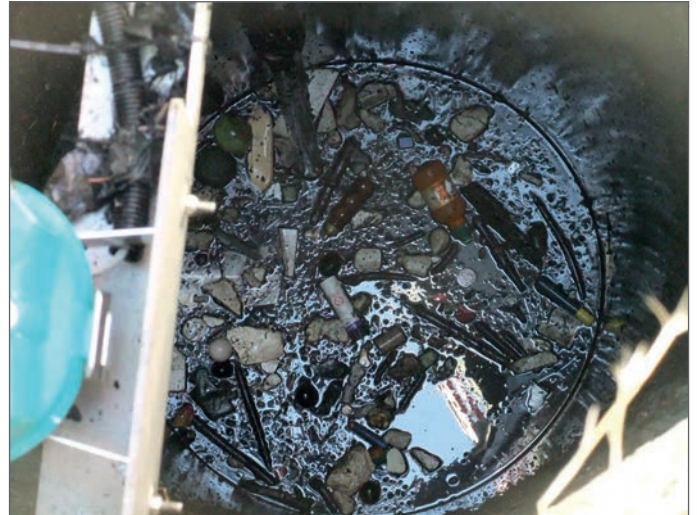
Floatable debris captured by the Downstream Defender®
