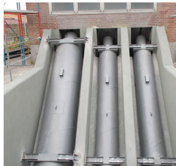
Kuhn Archimedean Screw Pumps
