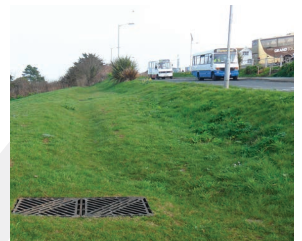
Retrofit infiltration, storage and control to mitigate flooding at a town car park
