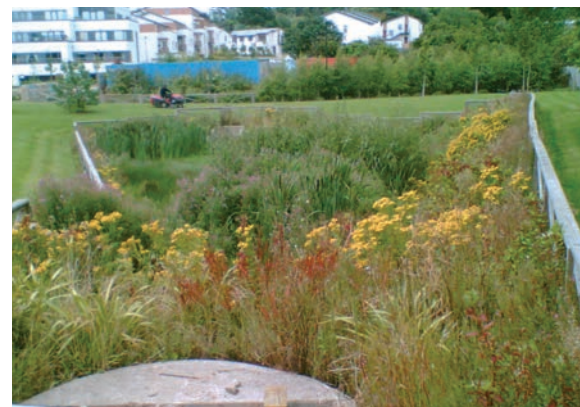
Protect - a stormwater storage area with pre-treatment
