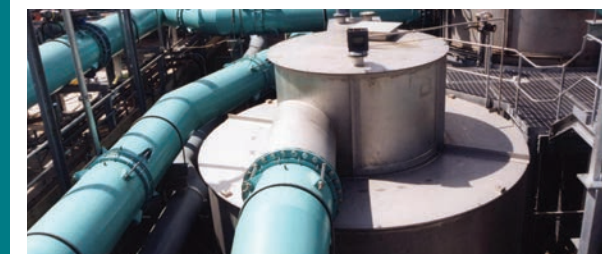
Hydrodynamic vortex grit removal
