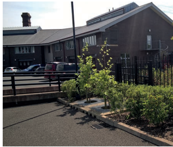
Biofiltration in a small-footprint and enhancing biodiversity
