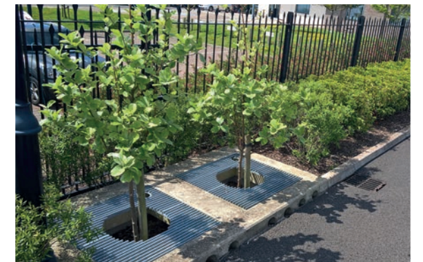
Small footprint stormwater treatment
