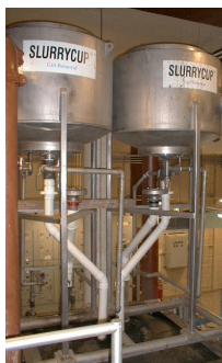
Gurnee and Clavey's Sludge Degritting Systems After Initial Start-up in 1998
