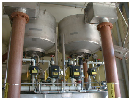
Gurnee and Clavey's Sludge Degritting Systems After Initial Start-up in 1998
