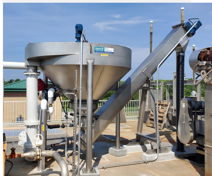
Gills Creek's Installed Hydro GritCleanse™ System
