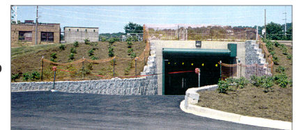
Entrance to underground facility where Storm King® units provide a sustainable solution for CSO treatment
