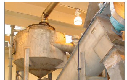
The Grit King® vortex separator removes sand and grit from the flow stream helping protect downstream infrastructure from wear and tear as well as clogging
