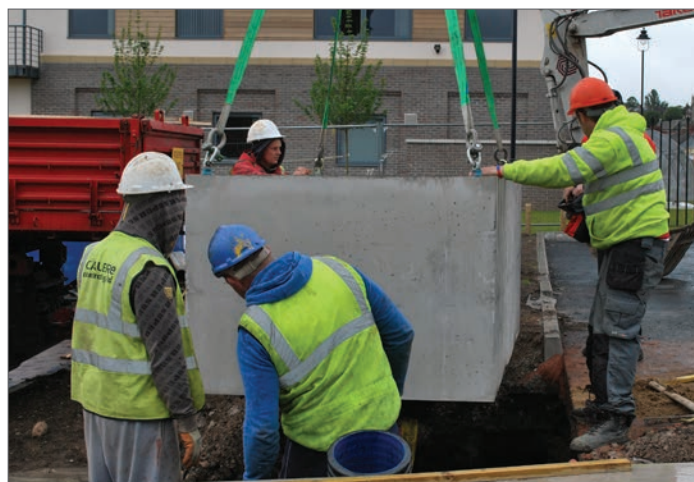
Chamber being lowered into position.
