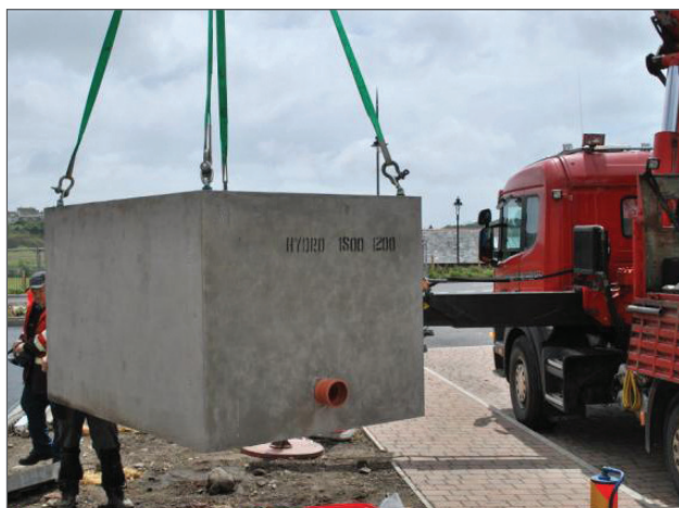
Chamber lift and correct lifting points.
