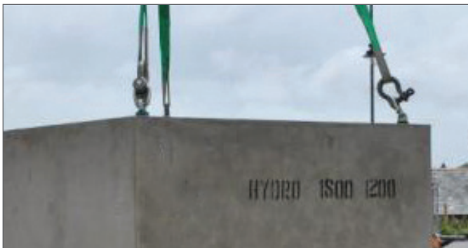
Example of lift and correct lifting points.
