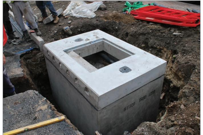
Bungs sealing the kerb inlet slots.
