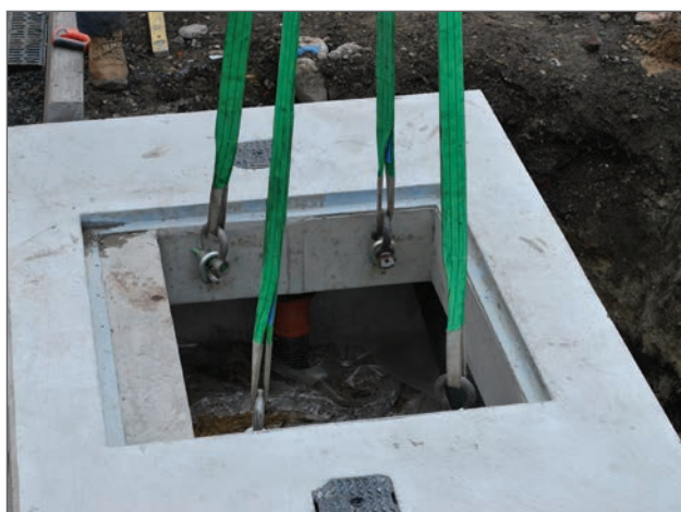
Cover lift and correct lifting points.
