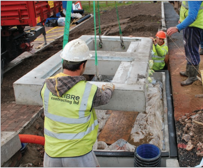
Chamber with Butyl sealant.
