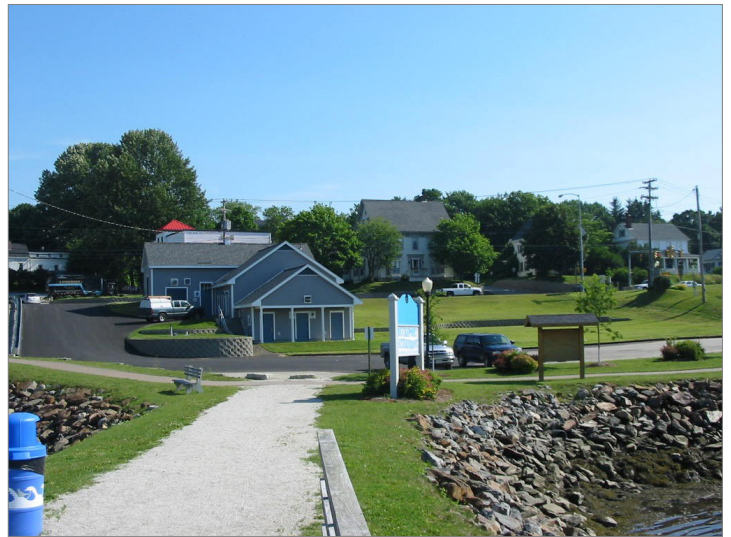
Bucksport CSO Facility From Fishing Pier
