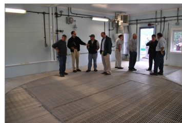
Interior Storm King® Facility
