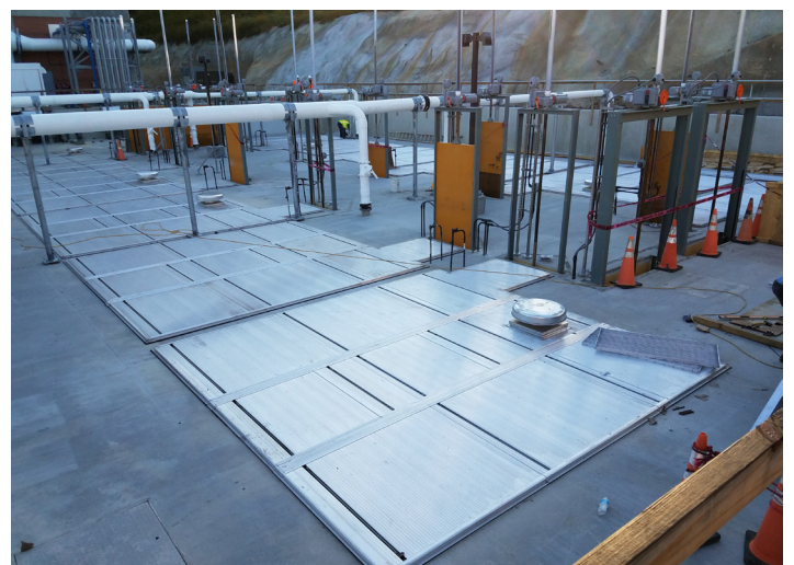
Installed In-Situ HeadCell® Tank Covers at RM Clayton Plant
