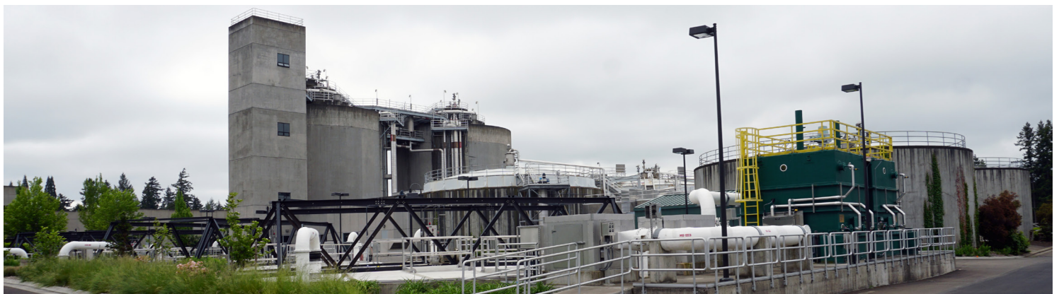
Rock Creek AWWTF
