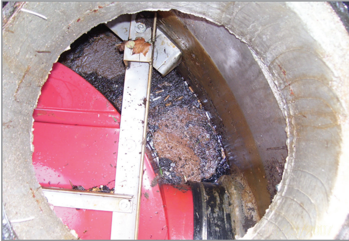
Fig. 2 The Downstream Defender® effectively captures and retains the bulk of solid pollutants from stormwater runoff, extending the maintenance life and performance of downstream retention ponds.
