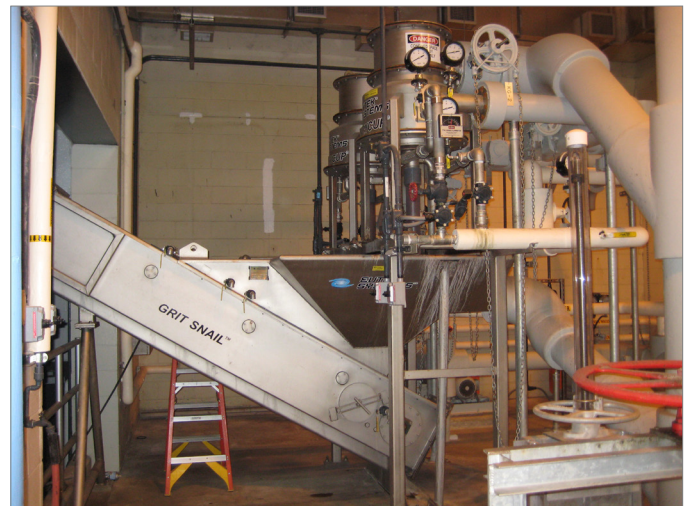
SlurryCup™ / Grit Snail® Grit Washing / Dewatering Systems at the Newton Plant
