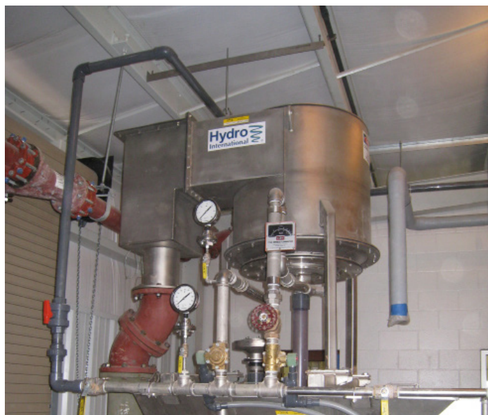
One of Tupelo Bayou's installed SlurryCup™ grit washing systems
