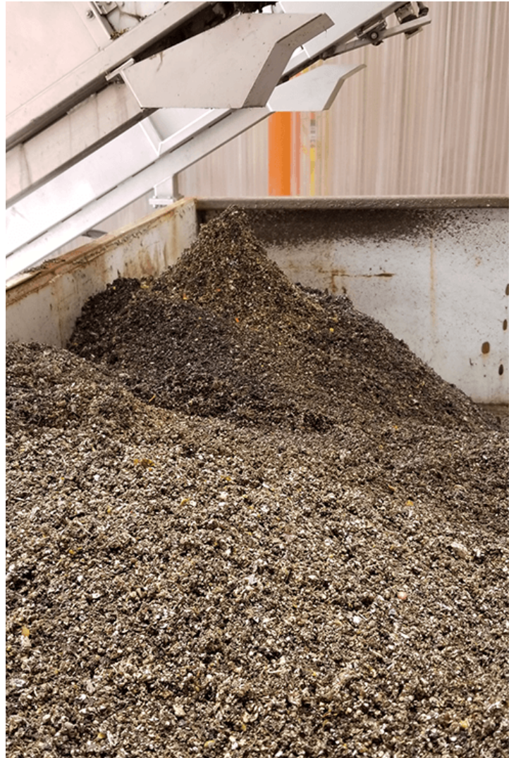
Airport WRF's Clean, Dry Grit Ready for Cost-Effective Disposal
